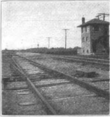
Derail Location and Tower
