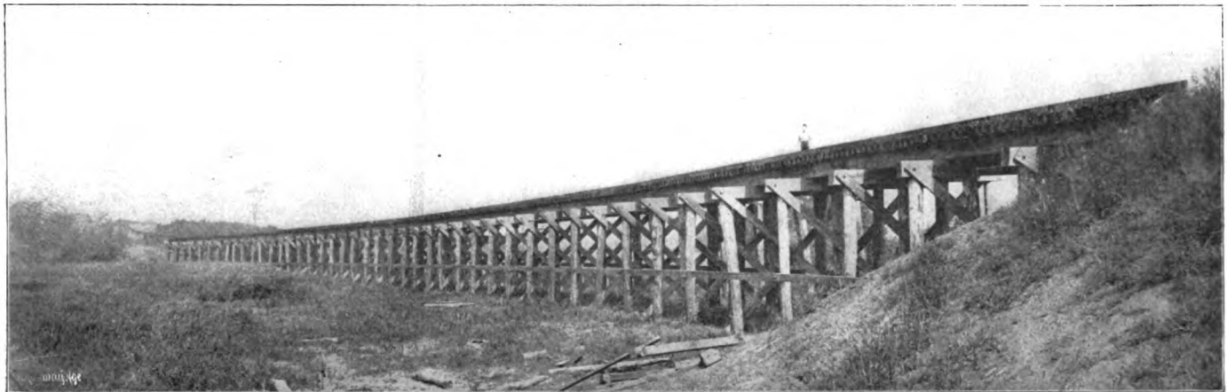
TOLEDO RAILWAY & TERMINAL COMPANY—TRESTLE OVER DUCK CREEK.
