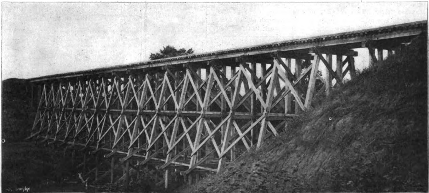
TOLEDO RAILWAY & TERMINAL COMPANY—TRESTLE OVER SWAN CREEK.
