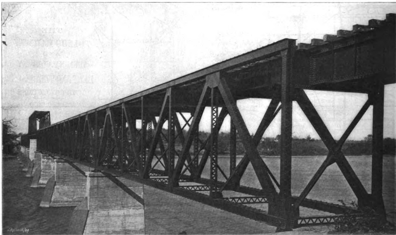
TOLEDO RAILWAY & TERMINAL COMPANY—UPPER BRIDGE, MAUMEE RIVER.
