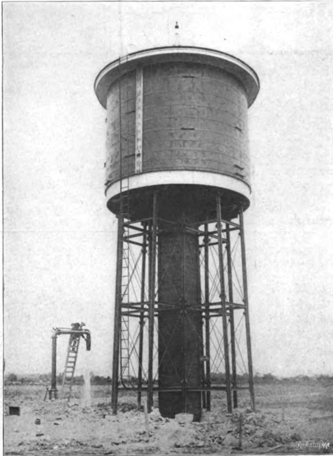
TOLEDO RAILWAY & TERMINAL COMPANY—WATER TANK.
